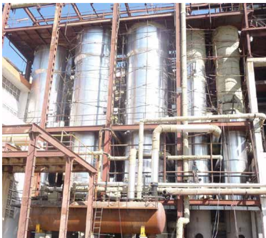
Figure 1. New falling-film evaporators and condensate tank during installation at ICPL
